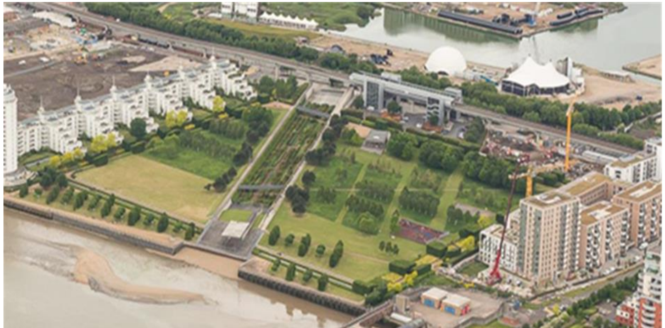
Thames Barrier Park
